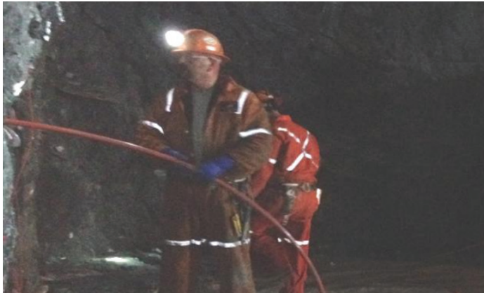
Operators charging the face.
