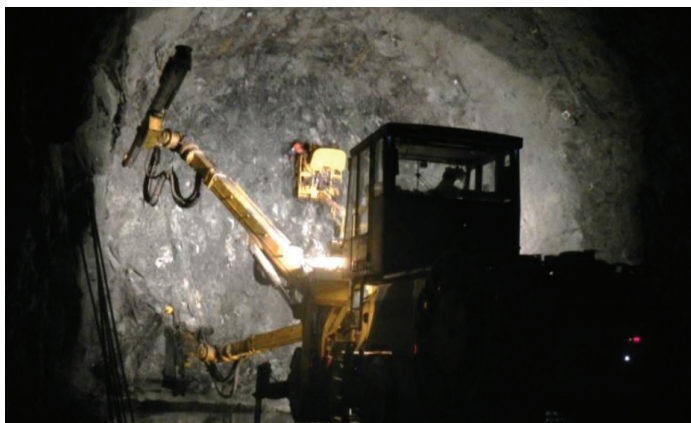
Jumbo drill in heading at Forrest Kerr.
