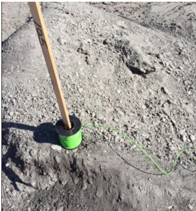
dynamic water. After the hole has been loaded, the wires are tied to a lath placed in the drill cutting pile. After stemming, the lath is moved closer to the hole so there is slack in the wire. The blaster has to go back periodically to check that there is still slack, as sometimes the wire gets pulled down the hole if slumping has occurred. If slack in the wire is not provided, wire breakage may occur.
