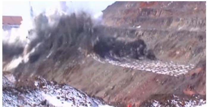
DIFFERENTIAL ENERGY technology allowed the operators to adjust the explosive energy in each hole based on the geology.
