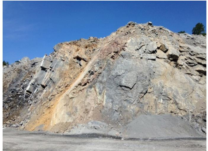
On shot day, the blast kept all of the rock inside the quarry and no objects flew up to the plant and administrative building directly opposite the angle holes. This shot also gave the quarry a shorter route to get to the crusher which should increase production.
