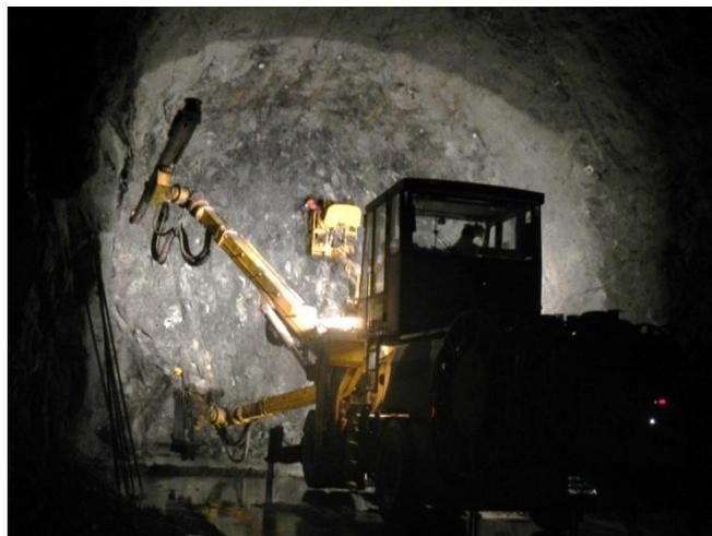
Initially a smaller 5 x 6m relief tunnel was conventionally blasted in the top middle section of the larger tunnel excavation.
