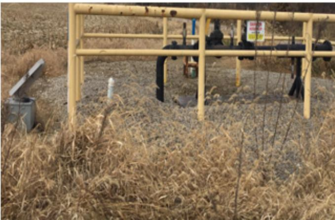
*Pipeline Riser and Permanent Seismograph*
